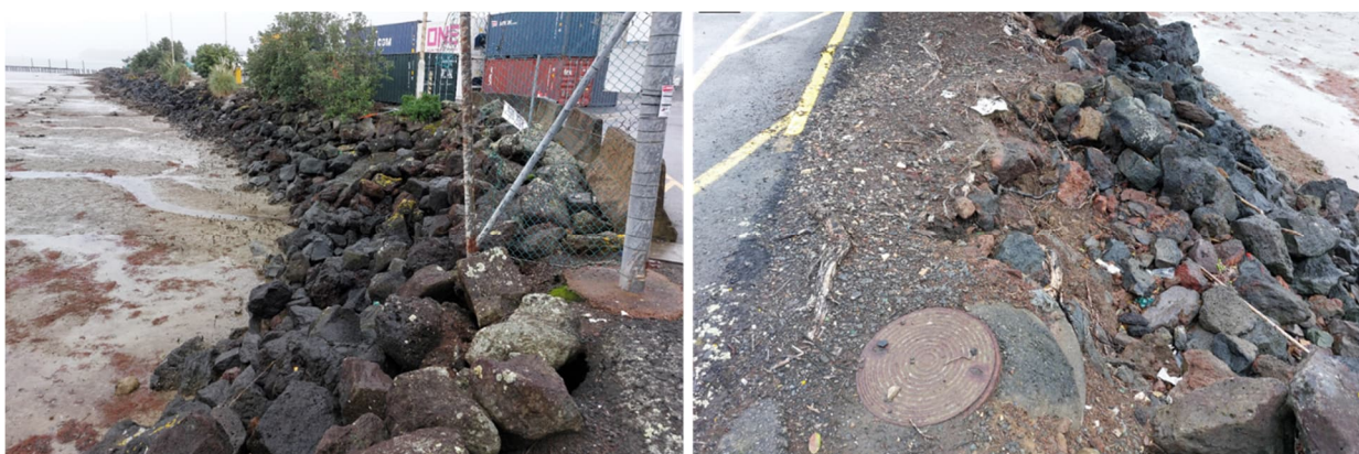
Photograph 2.2: Rock armoured edge of inner berthing area.
